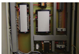
Fig. 16. Original wired M-S/TP system
